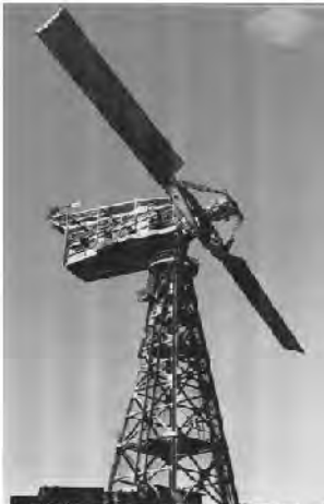
The world's first megawatt-size wind turbine near Grandpa's Knob Summit, Castleton, Vermont.
