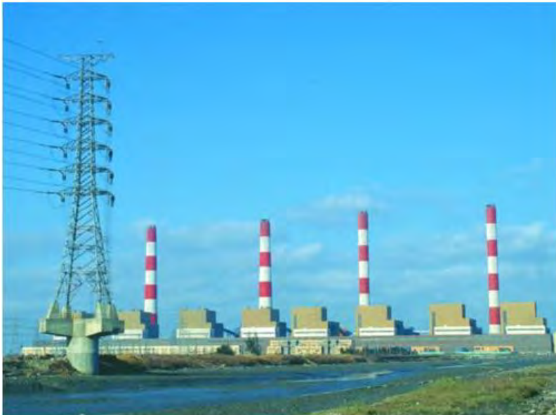
Taichung Power Plant
