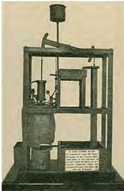
The model Newcomen engine upon which Watt experimented
