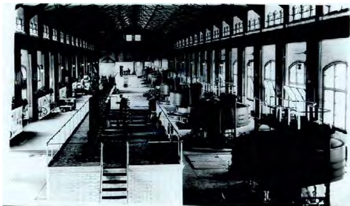
Power house 1, Niagara falls.
