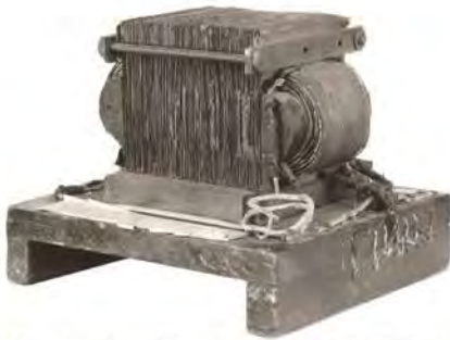
William Stanley's First Transformer built in 1885
